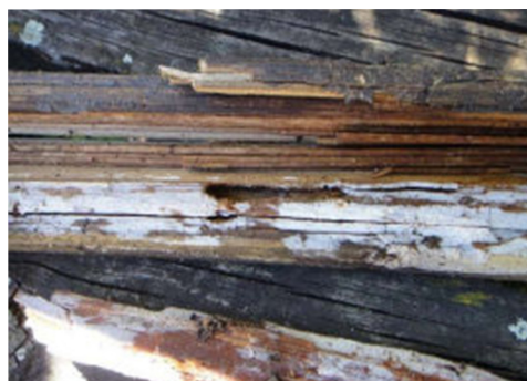
Figure 3b Roof construction of guest house with developed fruitbody of Hyphoderma setigerum
